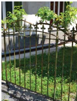
FERRONNERIE CLOTÛRE BLD ST PIERRE
